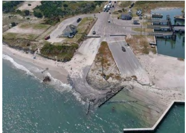
Chronic erosion has destroyed the vehicle stacking lanes and septic field at South Dock.
