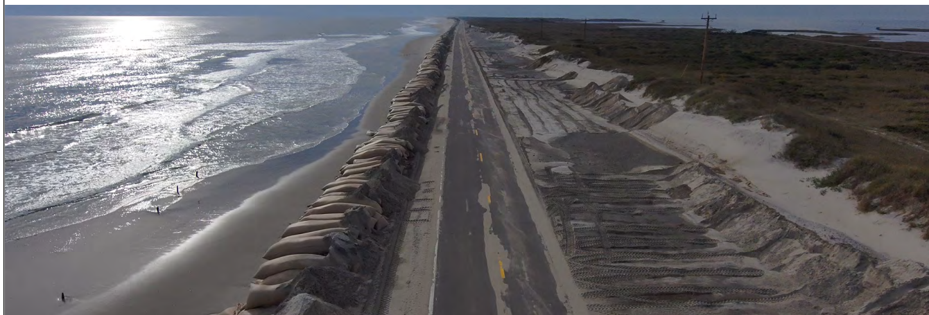
November 2024 drone footage illustrates the beach erosion, dune disturbance, and overwash continually impacting NC 12 on the Island in the wake of coastal storms.
