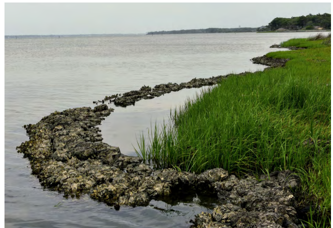
Shoreline restoration project with salt marsh plugs and oyster shells in Bogue Sound, NC.
